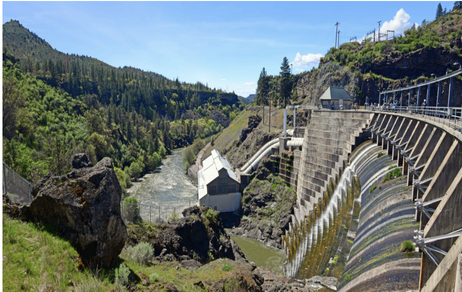
ONE OF THE FOUR HYDROELECTRIC DAMS SCHEDULED FOR REMOVAL AS PART OF THE KLAMATH RIVER RENEWAL PROJECT
